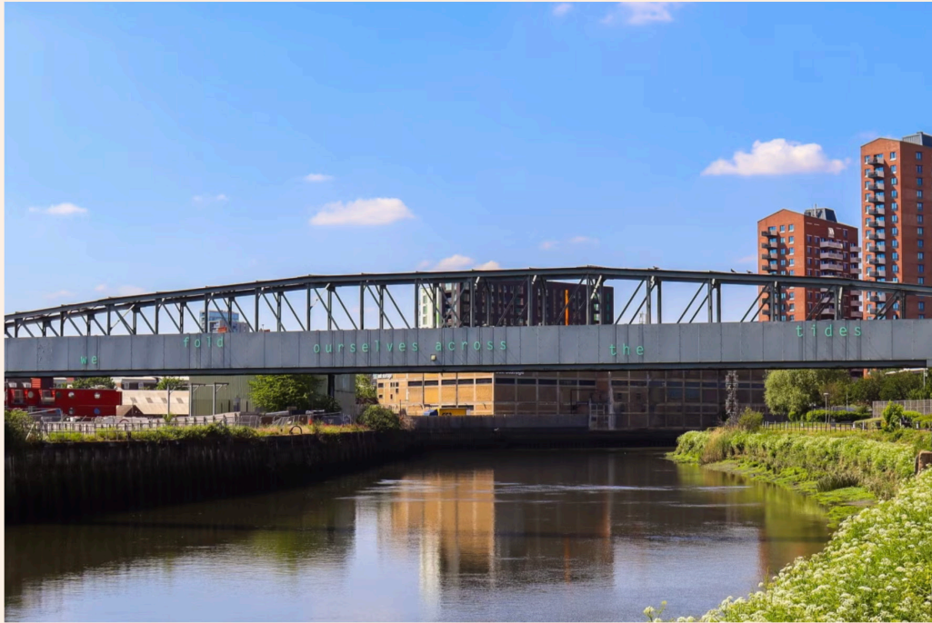
Connecting the London boroughs of Newham and Tower Hamlets, Helen Cammock's text-based 'On WindTides' is the latest addition to The Line
